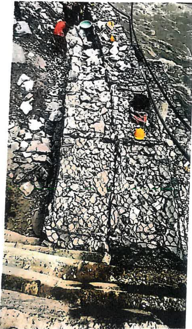
Construction of retaining structure/ Crate wall on left bank of river
